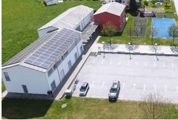
PV-Anlage MZH in Agarn
